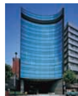
I-23 IKEBUKURO YS BUILDING 池袋YSビル
