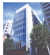
JRE Higashi-Gotanda 1Chome Building (Shinagawa-ku, Tokyo)
