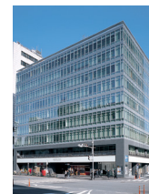
Sanno Grand Building
