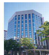
Daido Seimei Niigata Building (Niigata City, Niigata)
